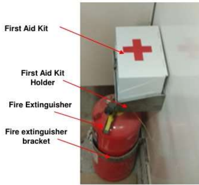
Figure 26: Fire extinguisher & First Aid Kit arrangement
