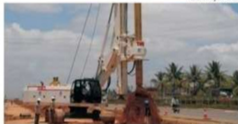
Hydraulic Piling Rig
