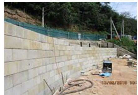
Figure 10 : Retaining wall: RDA SL
