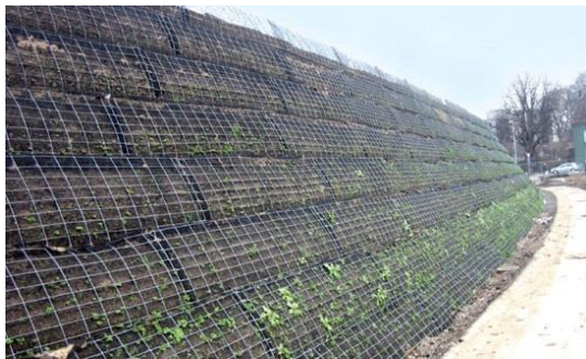
Fig 7: Geogrid application for slope protection: http://www.happho.com/geogrids-
