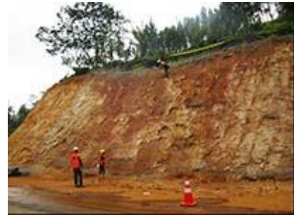
Figure 5: Modification of slope geometry: RDA SL
