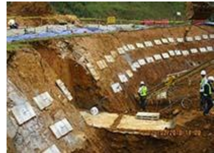
Figure 9: Rock bolting: RDA SL
