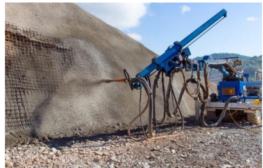
Figure 11: Shotcreting of slopes
