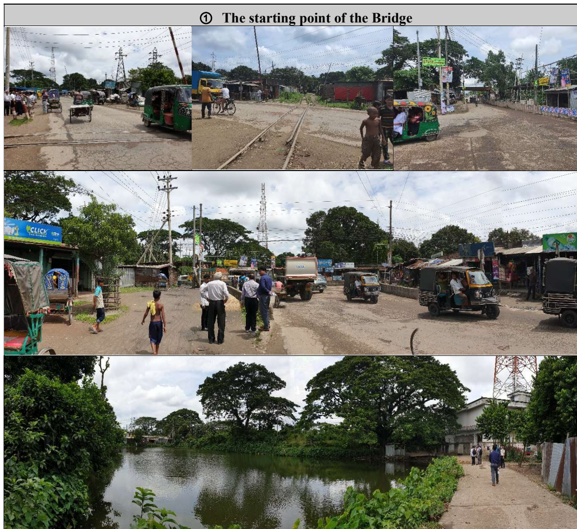
Figure 3-7 Starting Point of the Kewatkhalı Bridge
