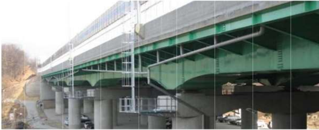
Figure 3-26 Example of Bridge Induction Drainage Treatment Method
