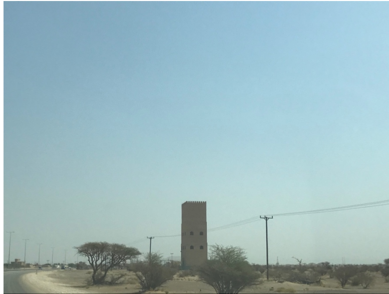
Figure 10-3 Water Tower Styled in Local Omani Tax Tower Design
