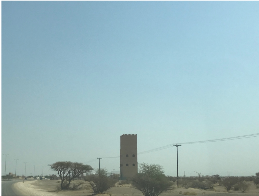
Figure 10-1 Water Tower Styled in Local Omani Design
