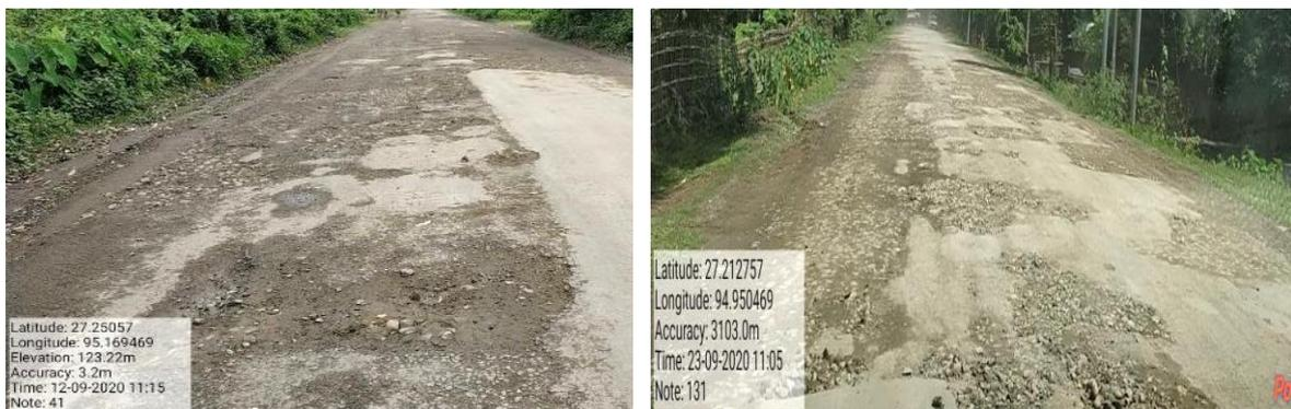
**Figure 1- 3: Photo of highly distressed road along stretch**
