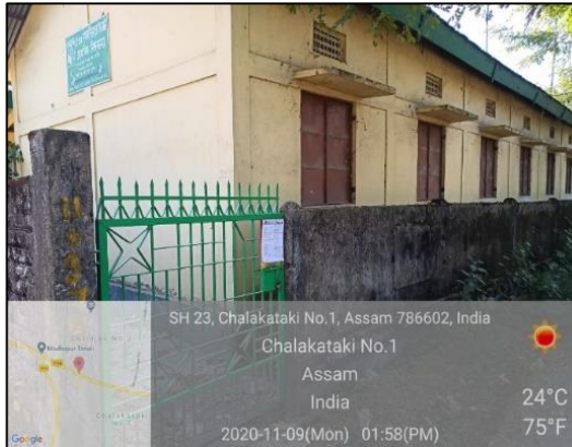
School building with boundary wall
