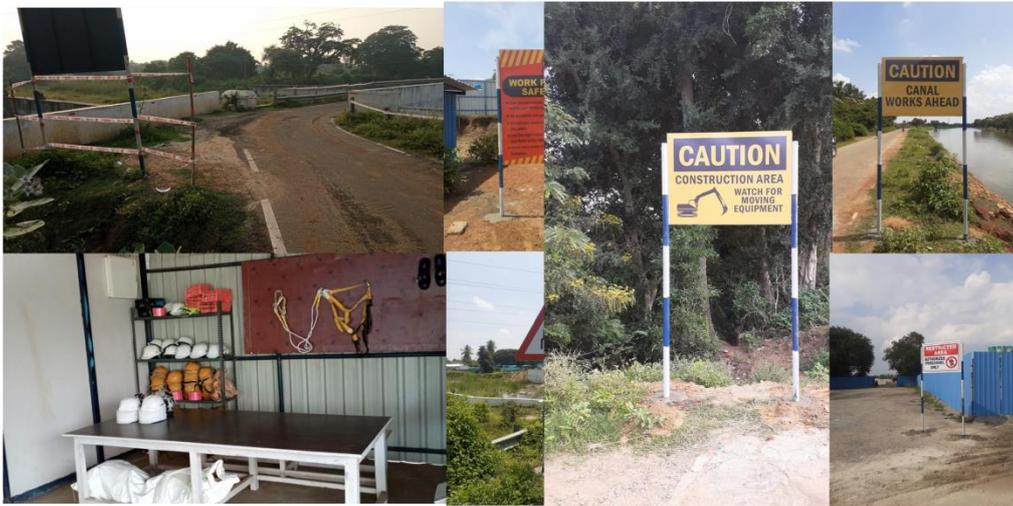
**Figure 9 : Display of caution boards in work site area**
