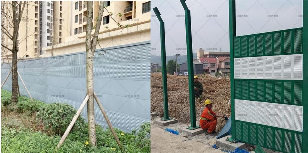
**Figure 6-10 Sound insulation fence recommended for construction site**
