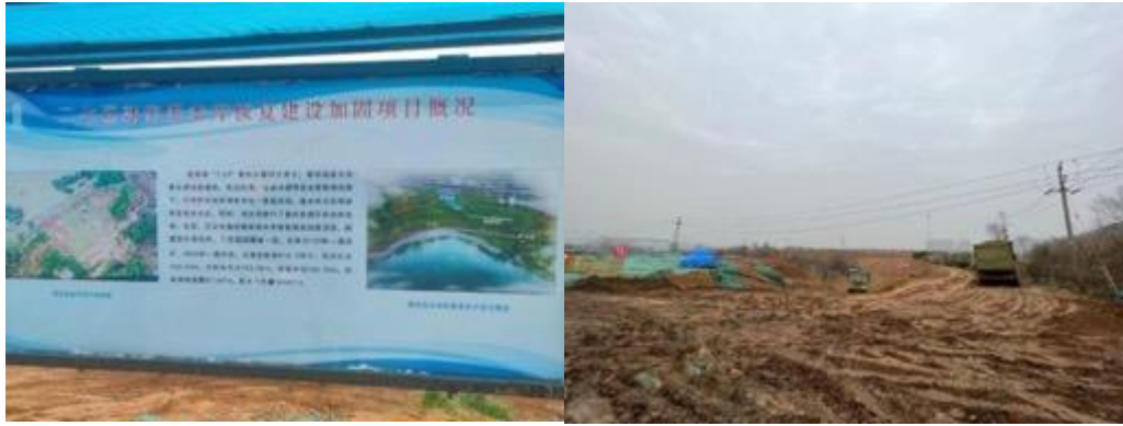
Figure 3-21 Construction site of Guojiazui reservoir restoration and construction reinforcement project (March 2022)
