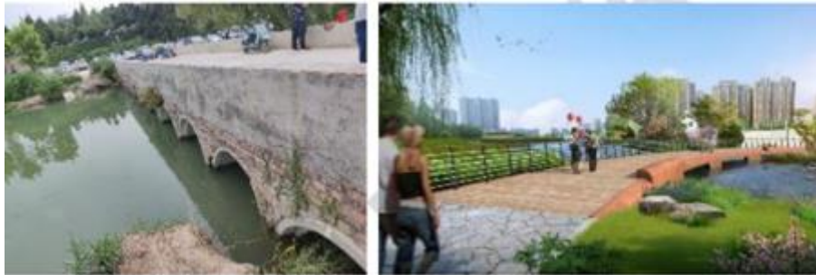
Figure 3-10 Before and after scheme of the south side bridge of the south water transfer
