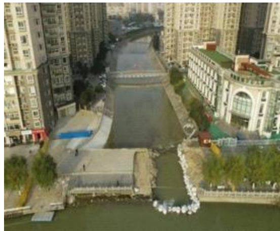
Figure 3-7 Damage to Binhu North Road Bridge
