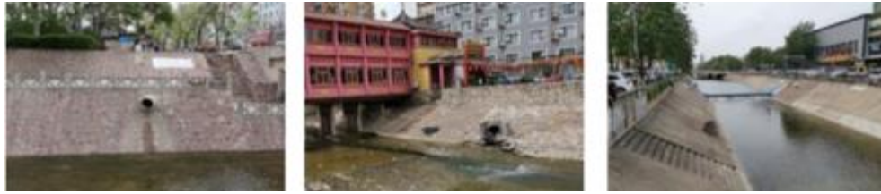
Figure 4-3 Part of the mixed flow outlet along the Jinshui River and the sewage pipeline in the river
