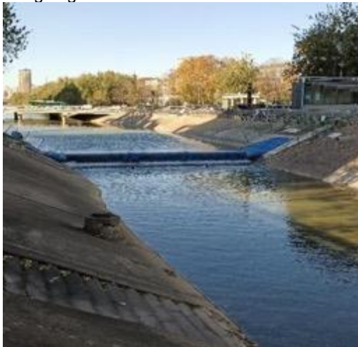
Zijingshan Road downstream barrage
