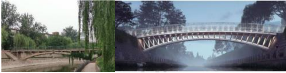
Figure 3-13 Pedestrian bridge on the east side of Chengdong Road before and after the project
