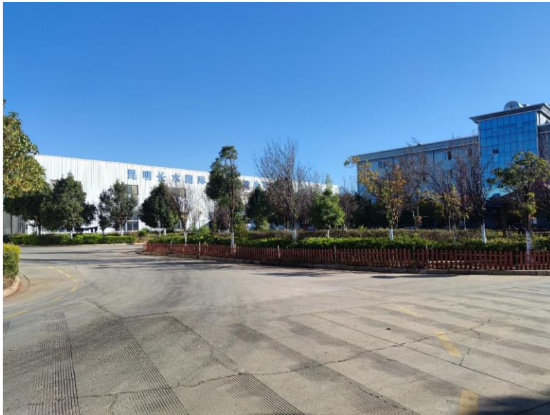
Fig. 4 Overview of domestic waste treatment station
