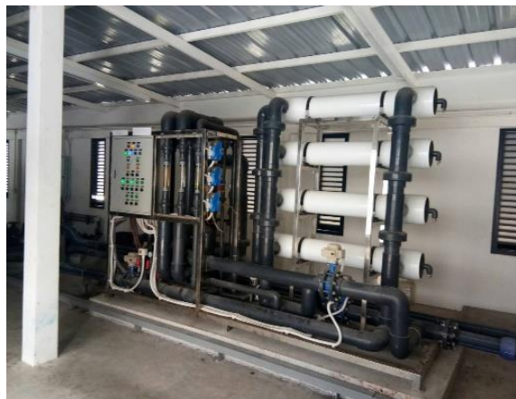
Figure 3.7 □ 33 RO water filtration system is located behind Terminal 2.
