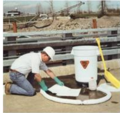
Figure 7 - Fuel/chemicals emergency prevention and clean-up kits will always be available at construction site.
