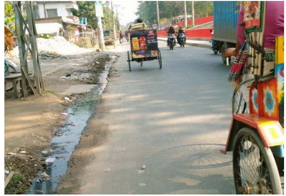
Figure 4.44 Roadside wasteful drainage, Rajshahi
