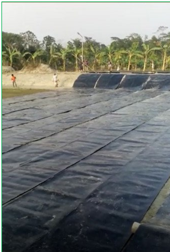
Figure 3.35 1.5 mm thick HDPE Liner on top of the Clay Layer shall be used to manage leachate
