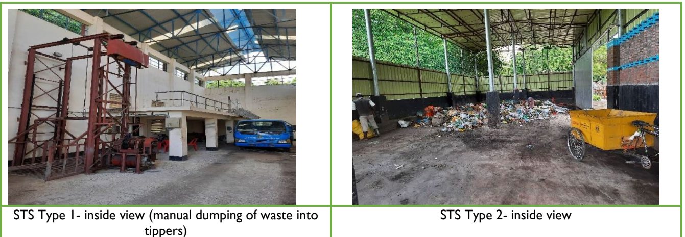
Figure 3.4 Example of Secondary Waste Storage for RCC Source: Consultant’s Team Site Visits and Field Surveys
