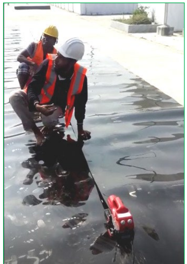
Figure 3.35 1.5 mm thick HDPE Liner on top of the Clay Layer shall be used to manage leachate
