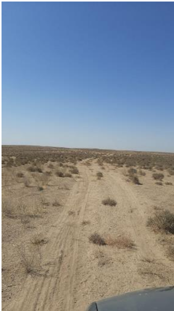
Figure 6-47. Road in Project Aol- 1
