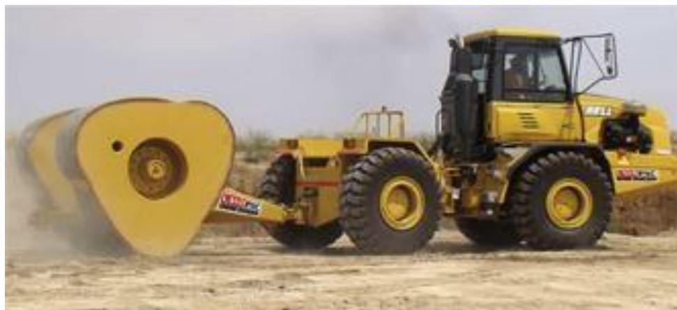
Figure 2-16. Rolling dynamic compaction (RDC)
