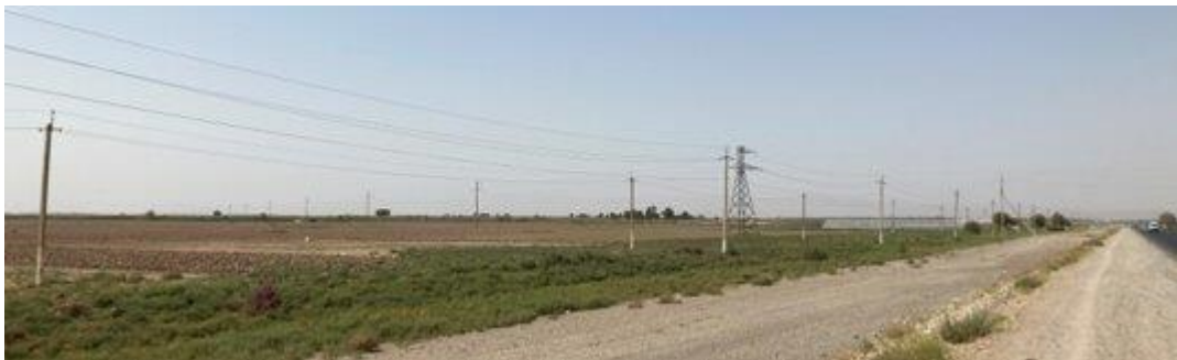
Figure 9-4. view 2 of typical farmland under the OTL
