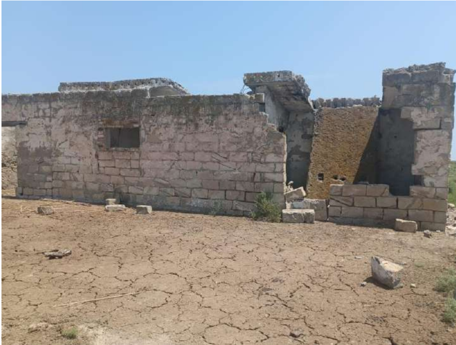
Figure 8-3 Military unused structure
