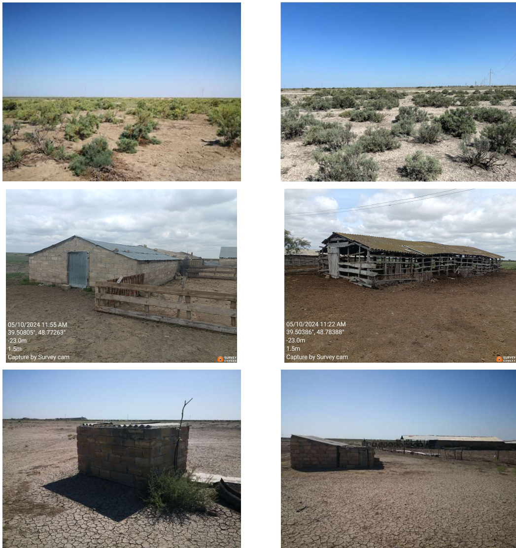
Figure 2-5 General Site Conditions and Existing Structures
