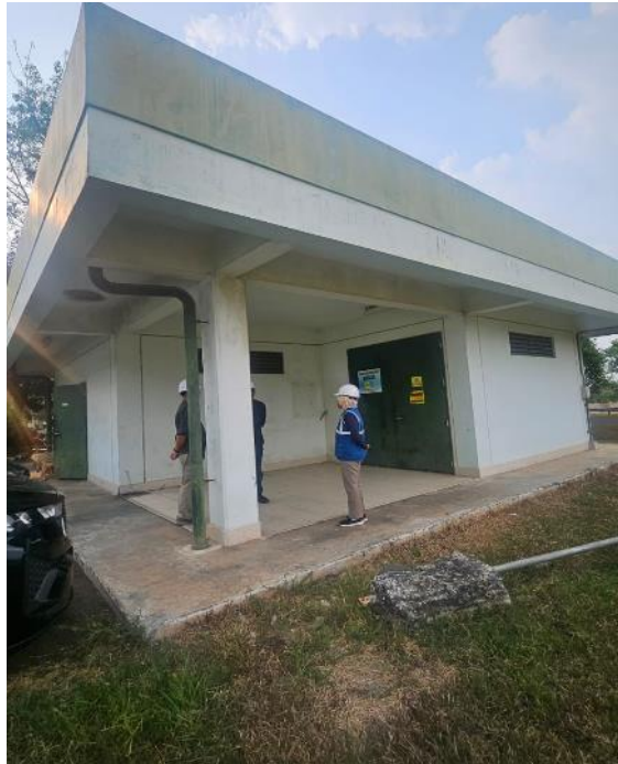
Distribution Substations Located in the Palembang Airport in UID S2JB.
