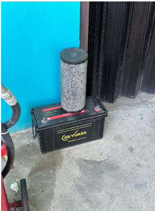
Improper storage of used battery in Banda Aceh warehouse in UID Aceh.
