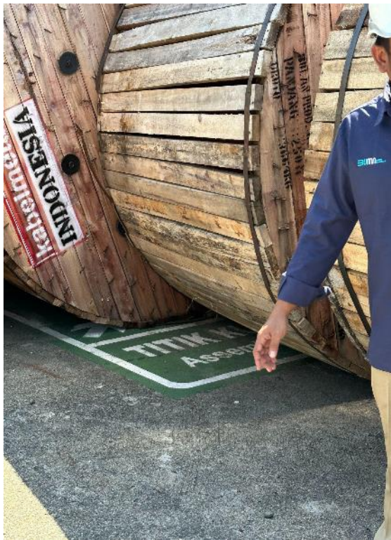
Occupied Assembling Point by cable materials in Banda Aceh warehouse in UID Aceh.
