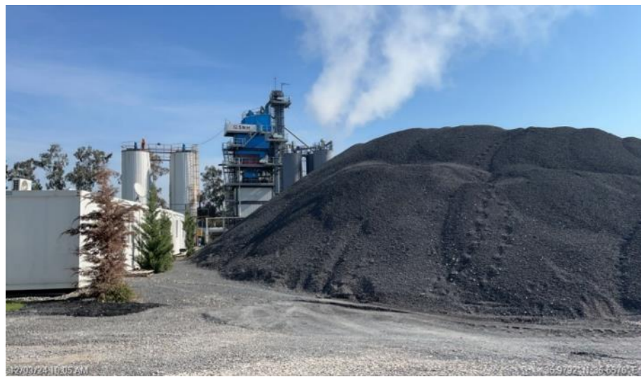
Figure 80. Asphalt Plant in Ceyhan Construction and Accommodation Site
