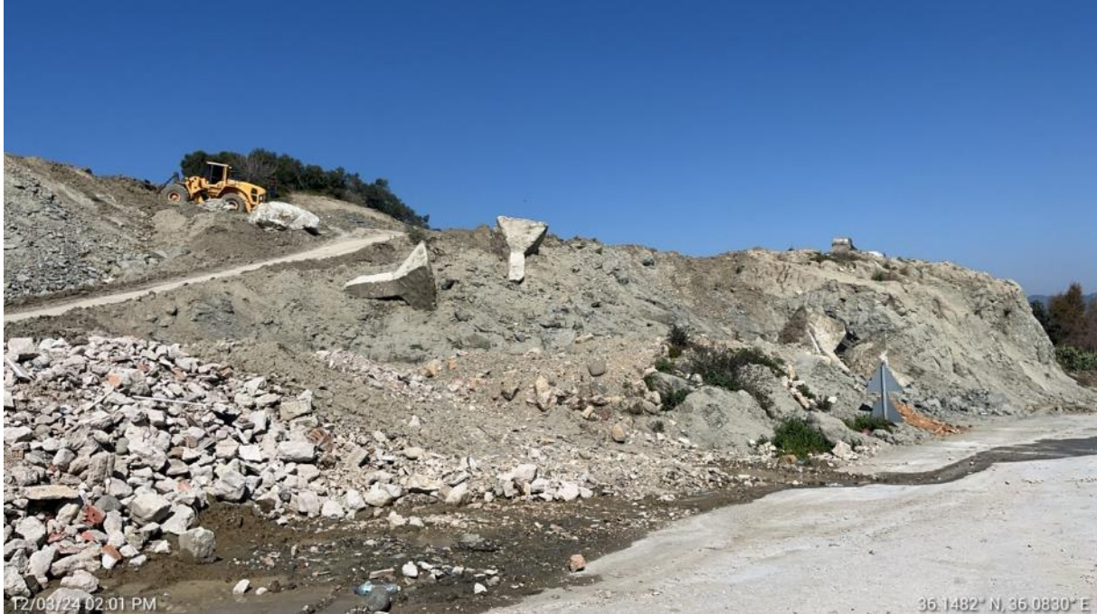
Figure 15. Landslide Removal Works
