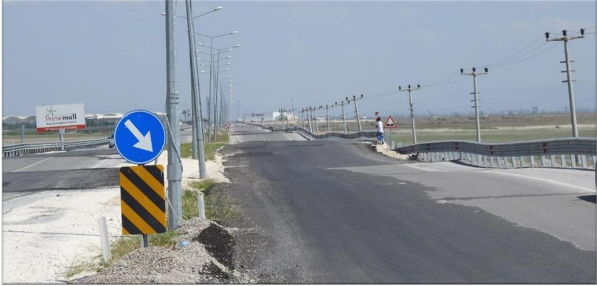
Figure 13. View of the Hatay Airport Road After the Earthquake (Km:2+840-3+480)
