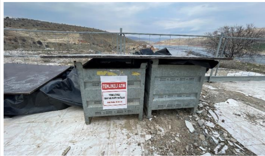
Figure 109. Hazardous Waste Containers in the Ağın Construction Site
