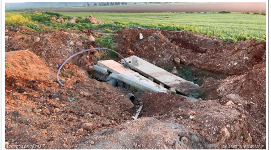
Figure 43. Old Septic Tank in the Kizilkaya Construction and Accommodation Site
