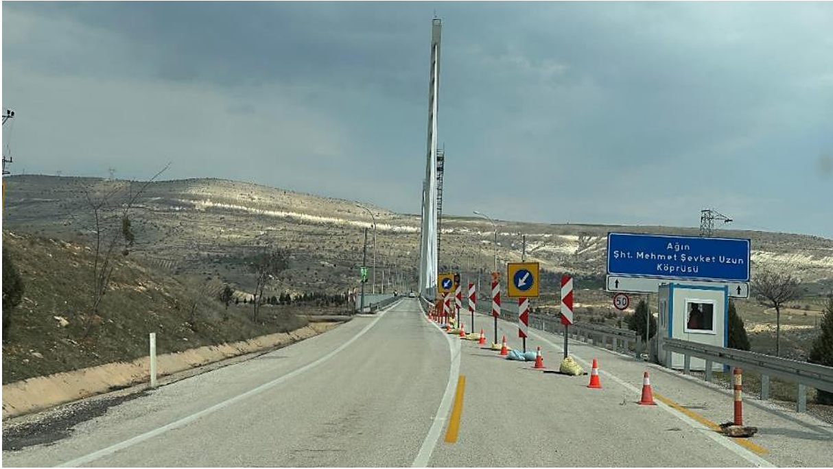
Figure 102. General View of Ağın Bridge -1
