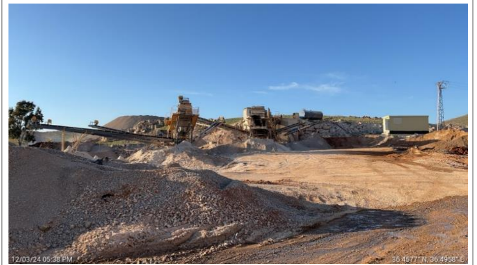
Figure 40. Crusher in Kizilkaya Quarry
