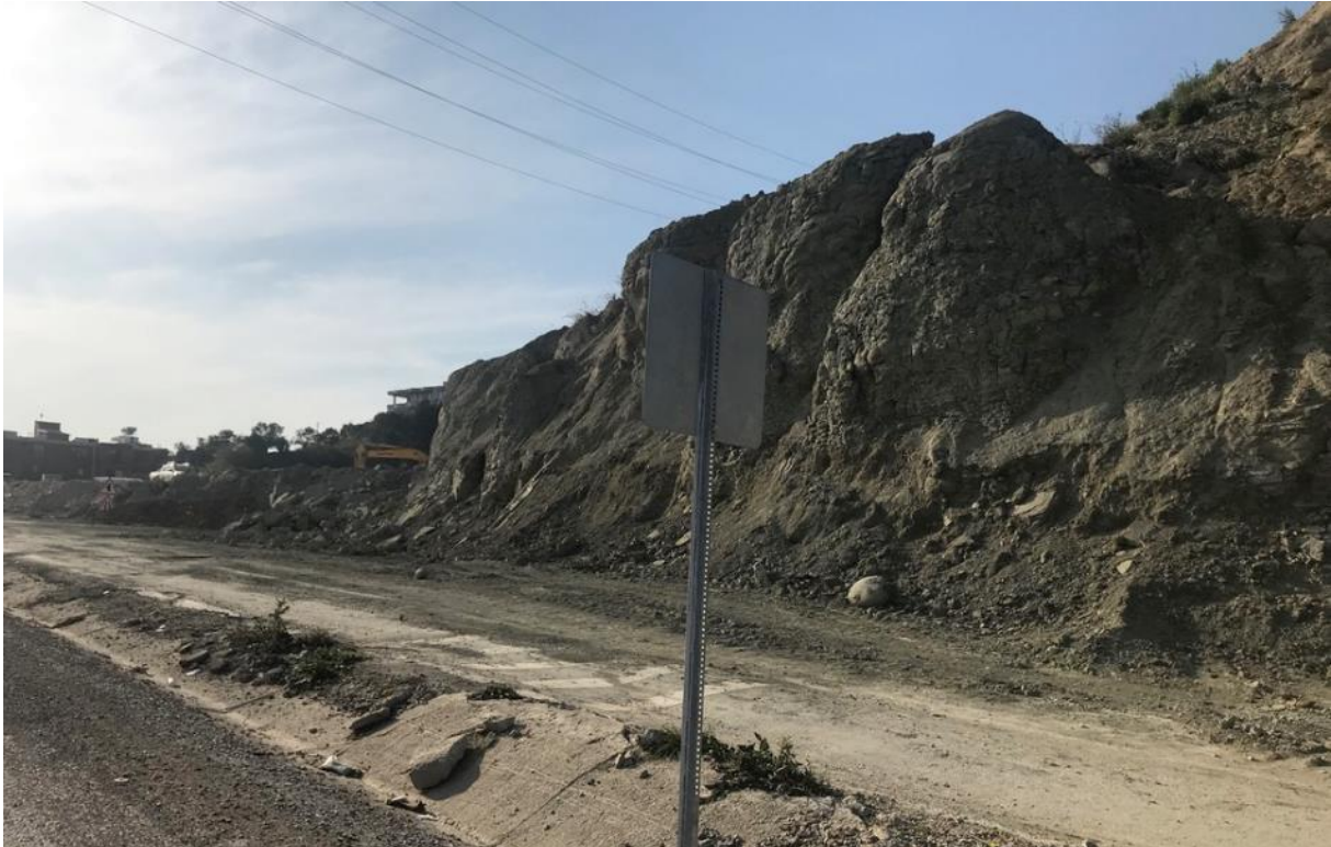
Figure 63. Landslide in Küçükkaracaay District Road
