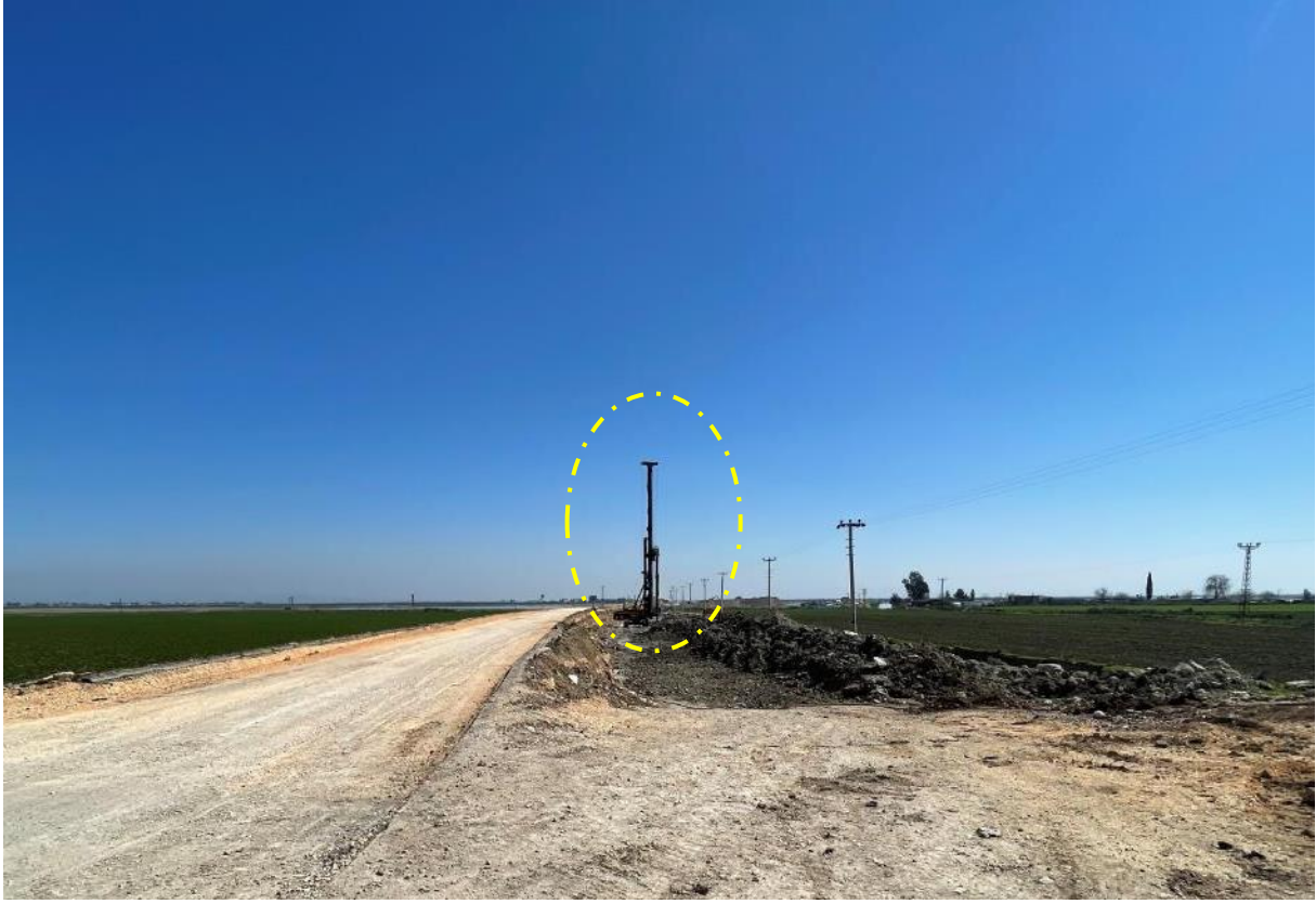
Figure 36. Deep Soil Mix (DSM) Machines on-site
