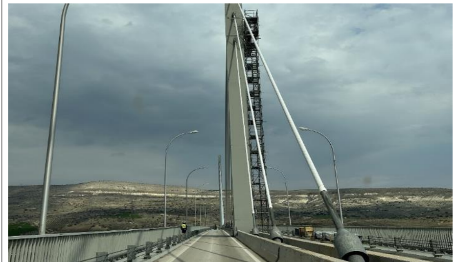
Figure 116. The scaffold set up at the Ağın Bridge
