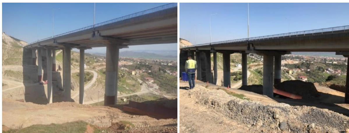
Figure 79. Başpınar Village and Başpınar Viaduct
