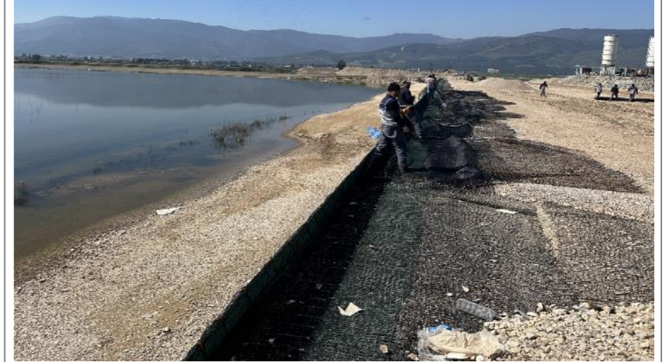
Figure 55. At the Hatay Airport Road Construction Site, Working at Heights
