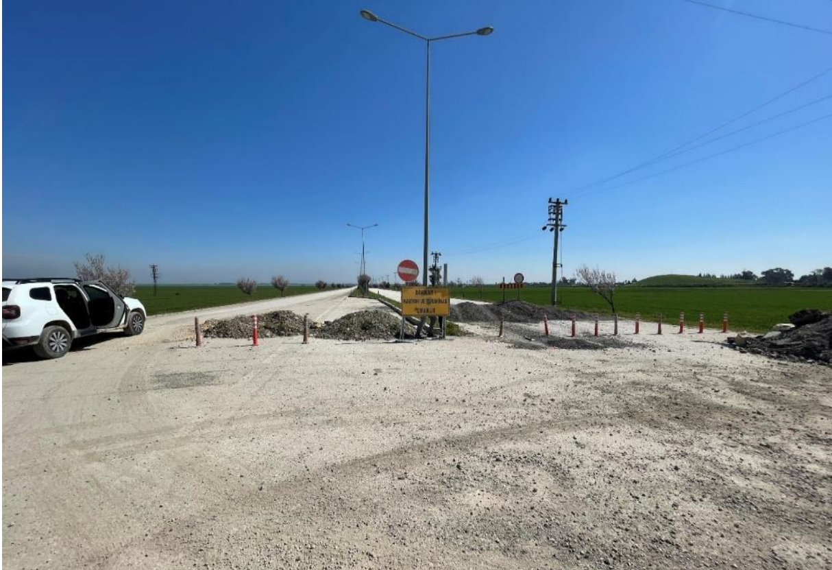
Figure 35. Entrance of the Sub-Project Construction Area
