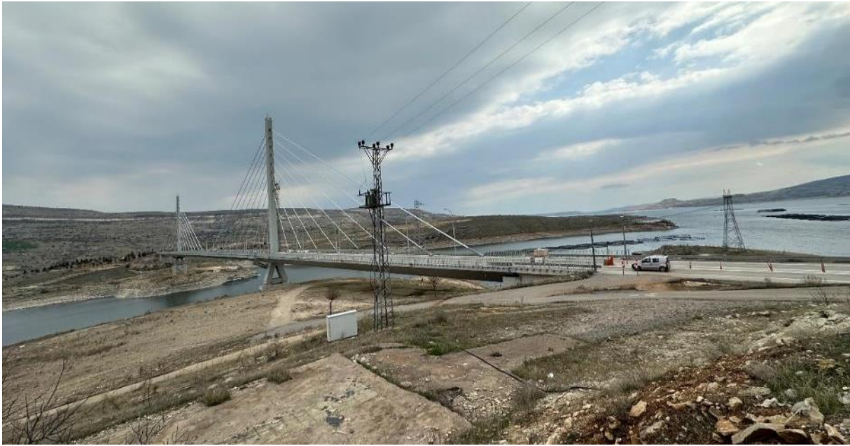
Figure 103. General View of Ağın Bridge -2
