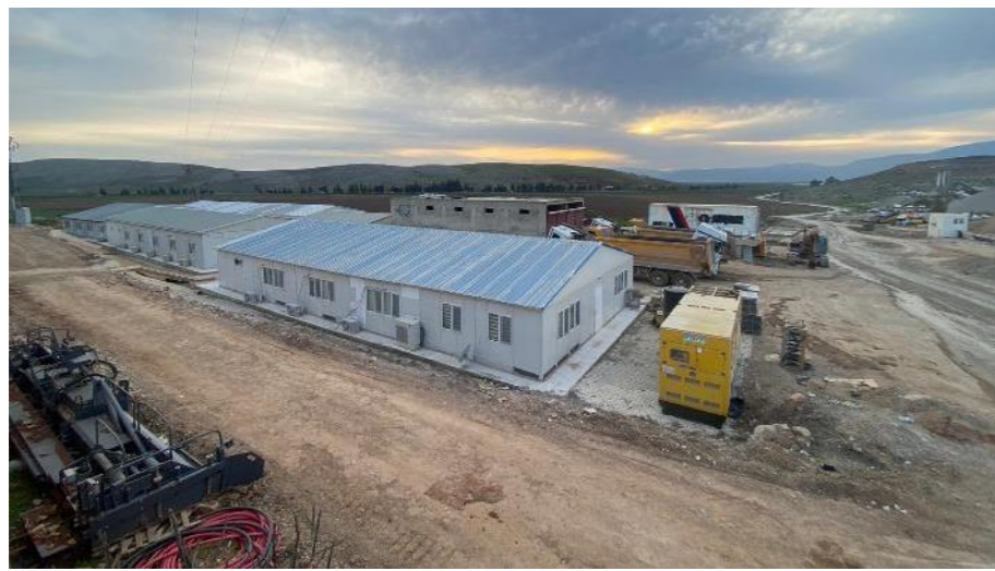
Figure 38. Kizilkaya Construction and Accommodation Site
