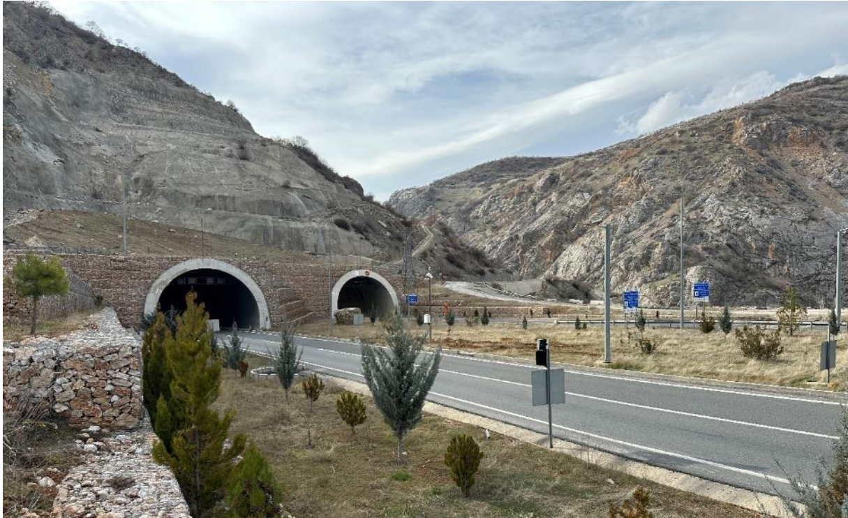
Figure 20. Erkenek Tunnel – Entrance Portal
