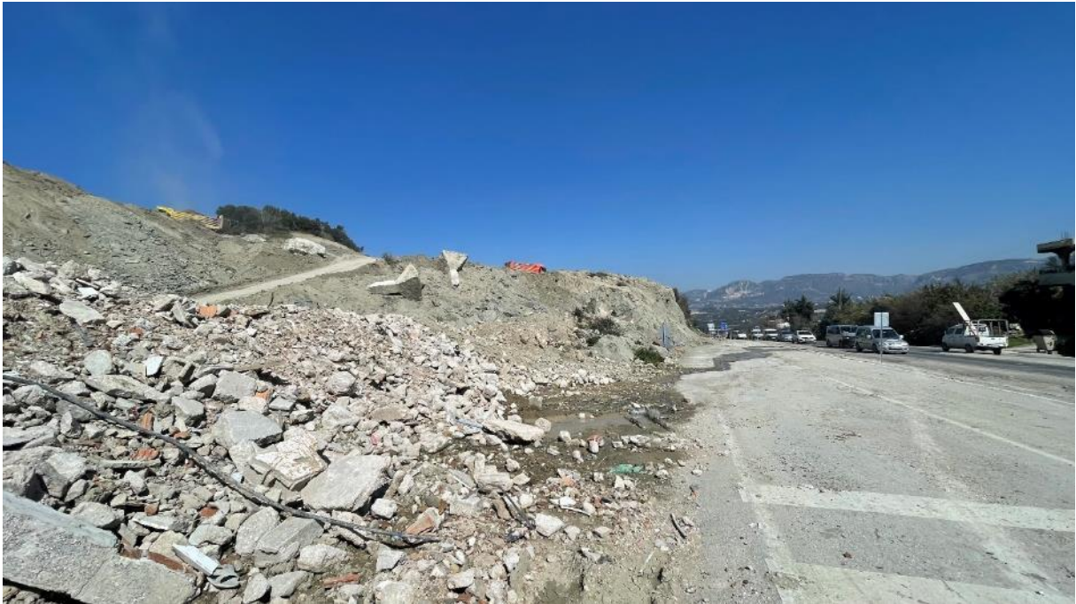
Figure 60. Landslide Removal Works at the Project Site
