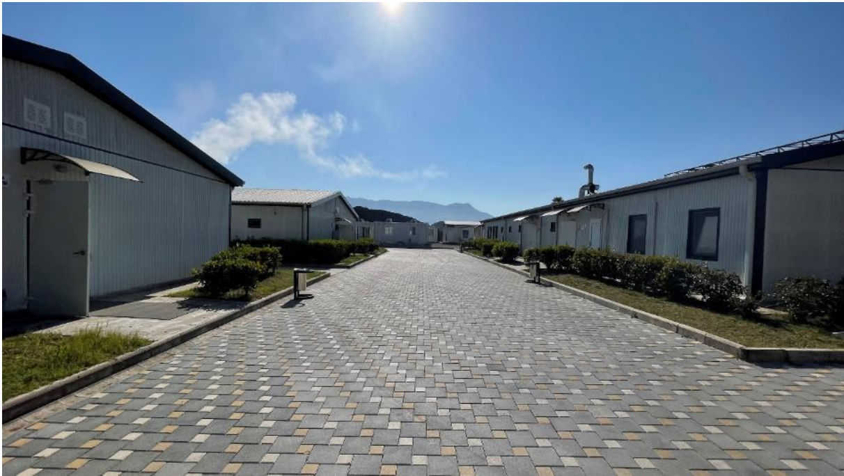
Figure 76. Ceyhan Construction and Accommodation Site - Accommodation Area
