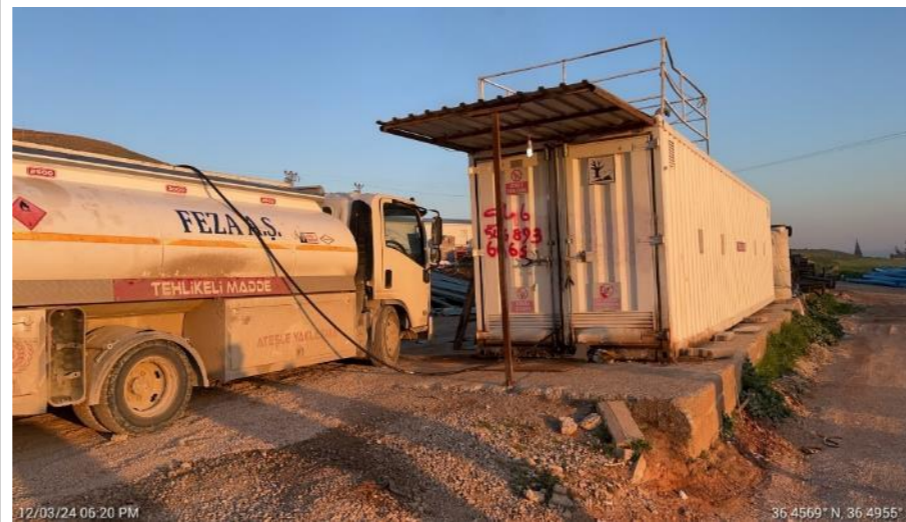
Figure 48. Chemical Storage Tank in the Kızılkaya Construction and Accommodation Site
