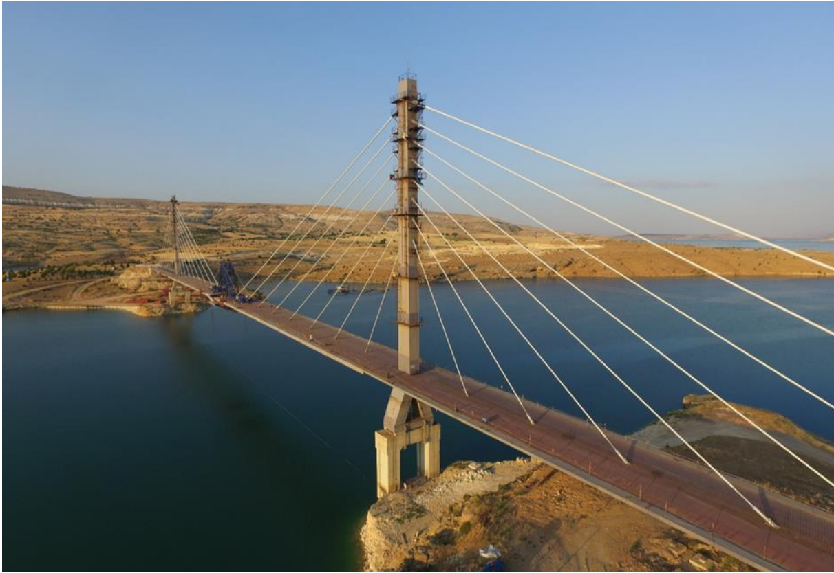
Figure 28. General View of Ağın Bridge
