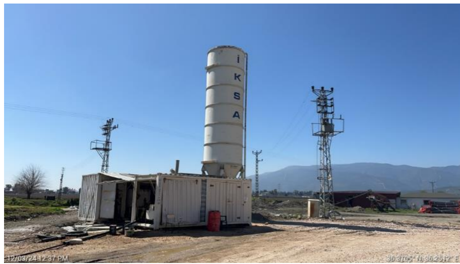
Figure 41. Deep Soil Mixing Station-1 at the Hatay Airport Road
