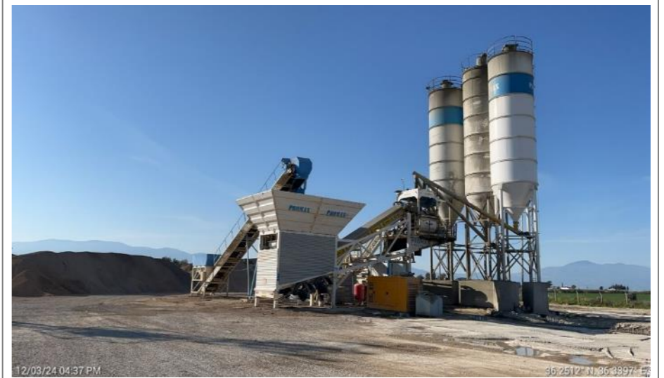
Figure 67. Concrete Plant used for Bridge Construction in Demirköprü
