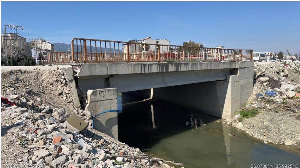
Figure 16. Bridge to be Reconstructed
