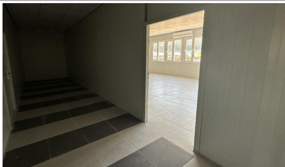
Figure 71. Office Building in Kuruyer Construction and Accommodation Area
