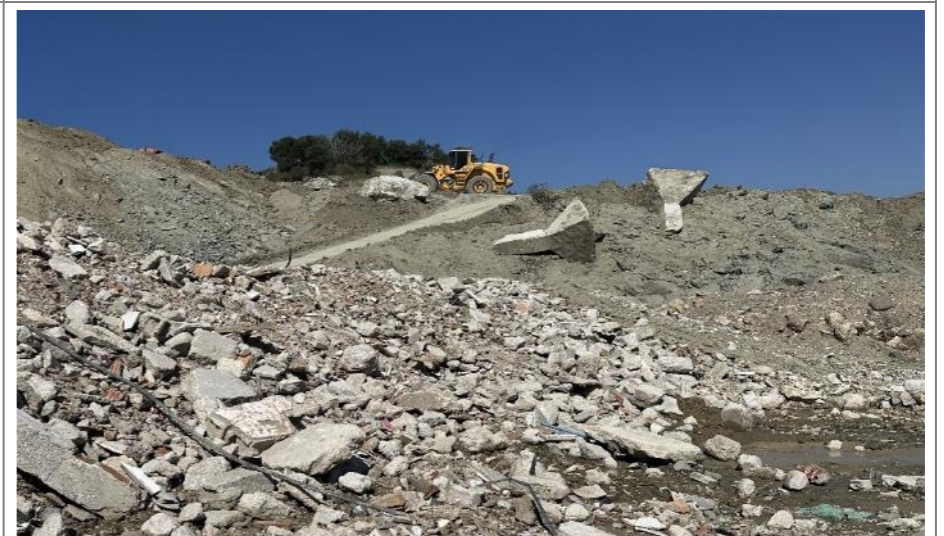
Figure 73. Landslide Area on the Antakya-Samandağ Road.
