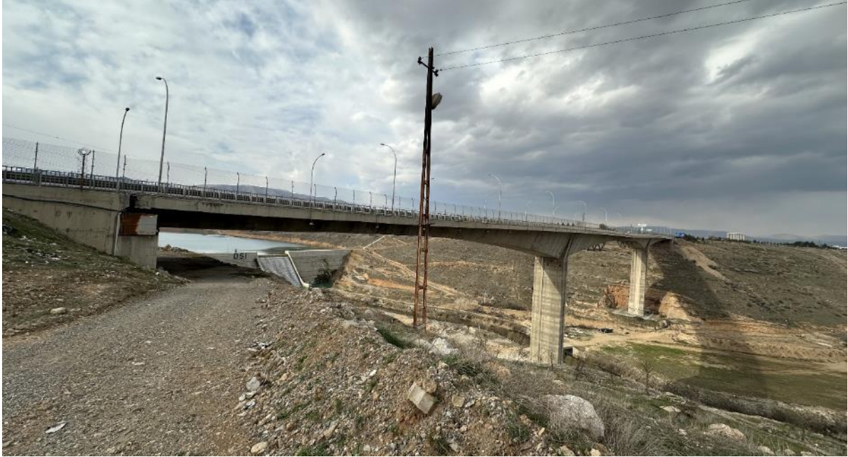
Figure 98. View of The Beylerderesi Bridge
