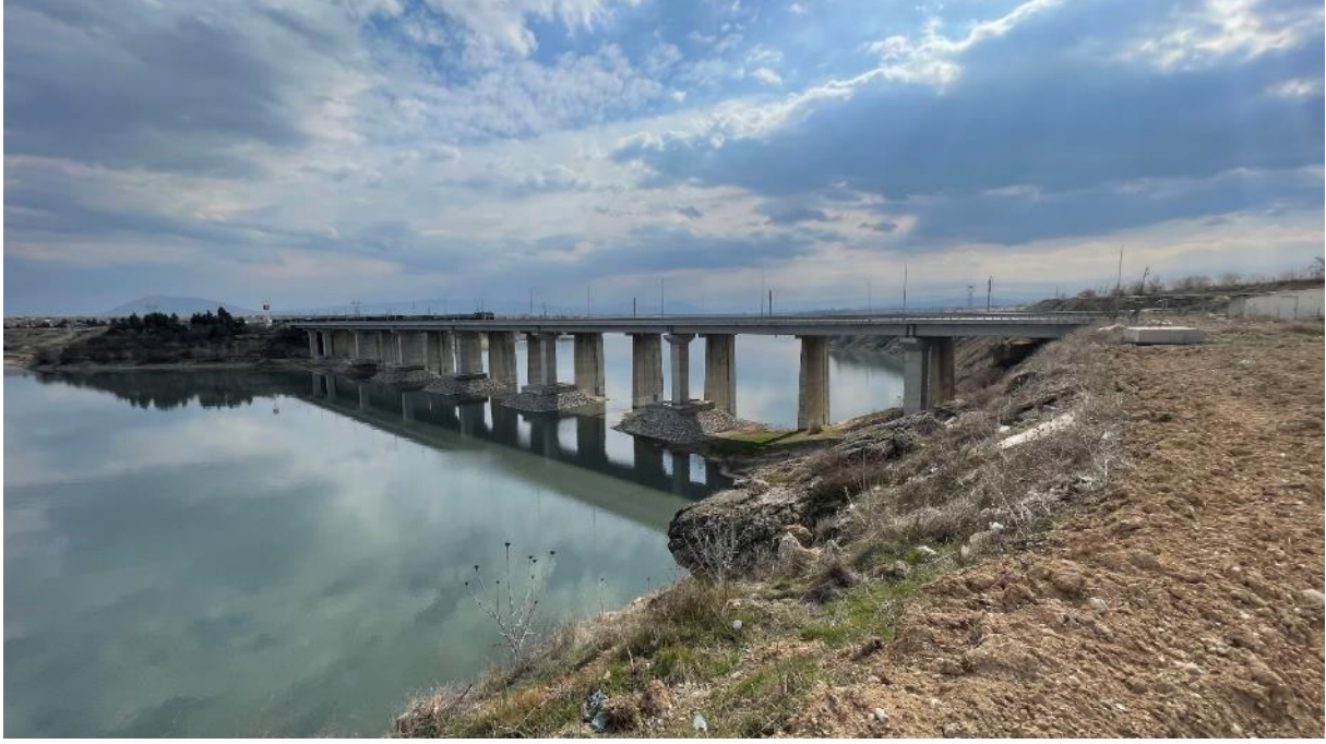
Figure 101. View of the Tohma Bridge
