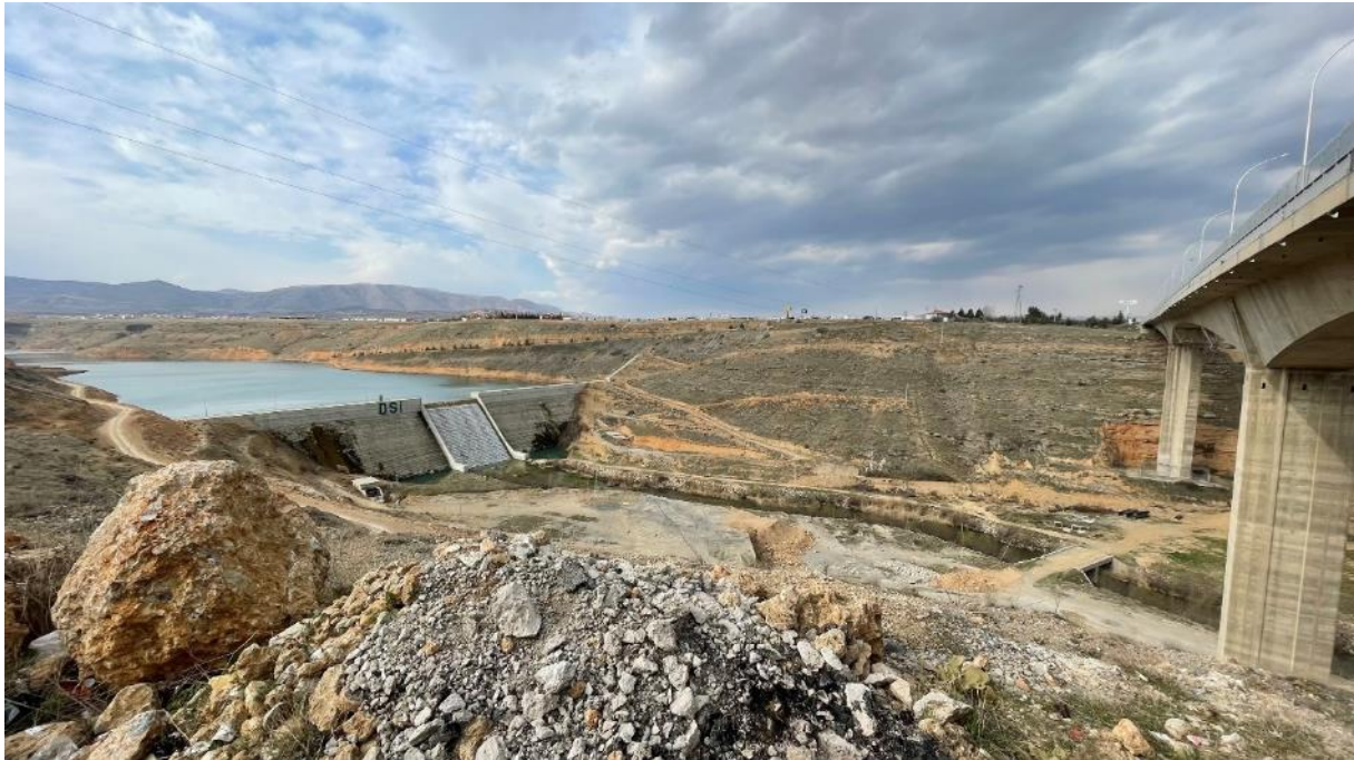
Figure 100. Yeşilvadi Reservoir and Beylerderesi Stream under the Beylerderesi Bridge
