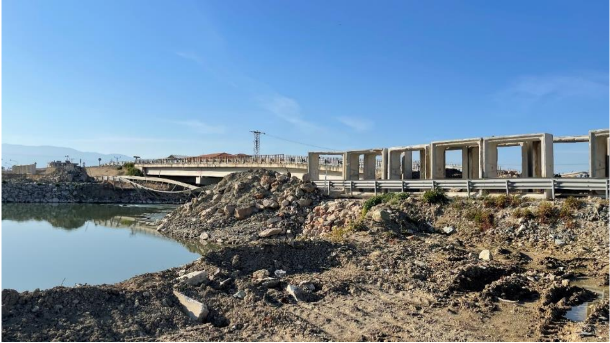
Figure 56. Demirköprü Bridge Construction Area
