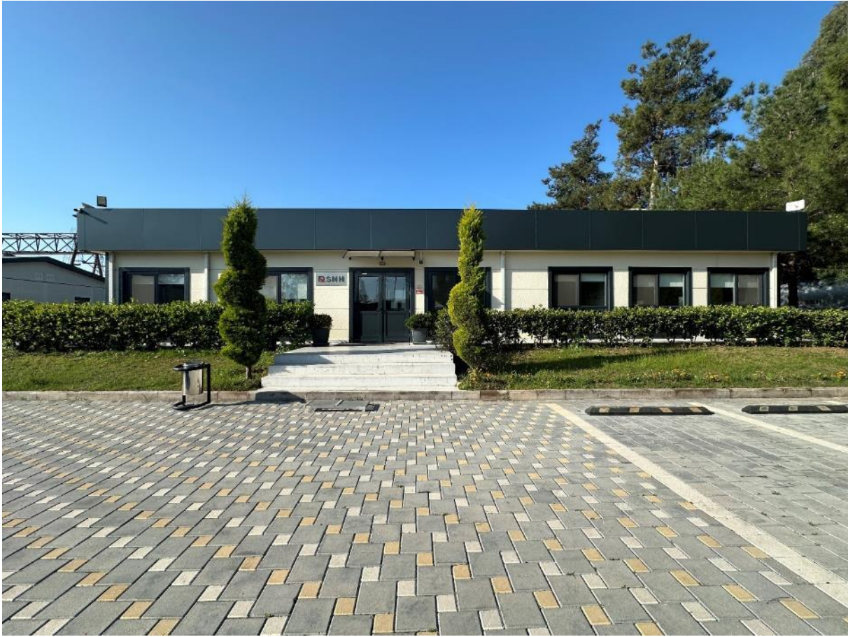
Figure 75. Ceyhan Construction and Accommodation Site - Offices
