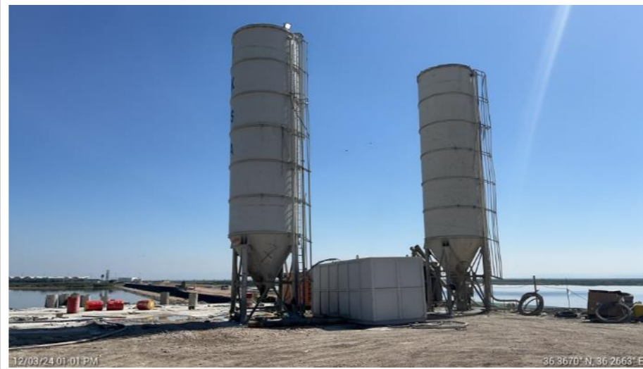
Figure 42. Deep Soil Mixing Station-2 at the Hatay Airport Road
