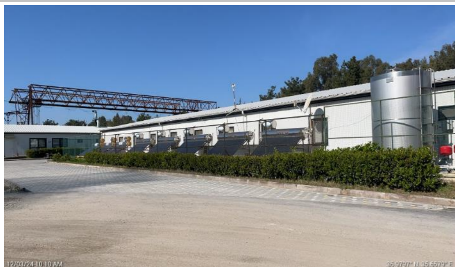
Figure 86. Solar Panels in Ceyhan Construction and Accommodation Site
