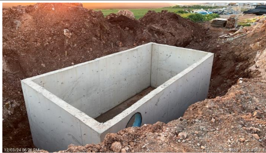
Figure 44. New Septic Tank in the Kizilkaya Construction and Accommodation Site
