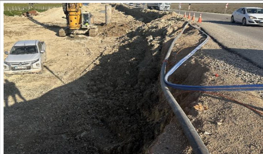
Figure 72. Antakya-Reyhanlı Road Construction Area
