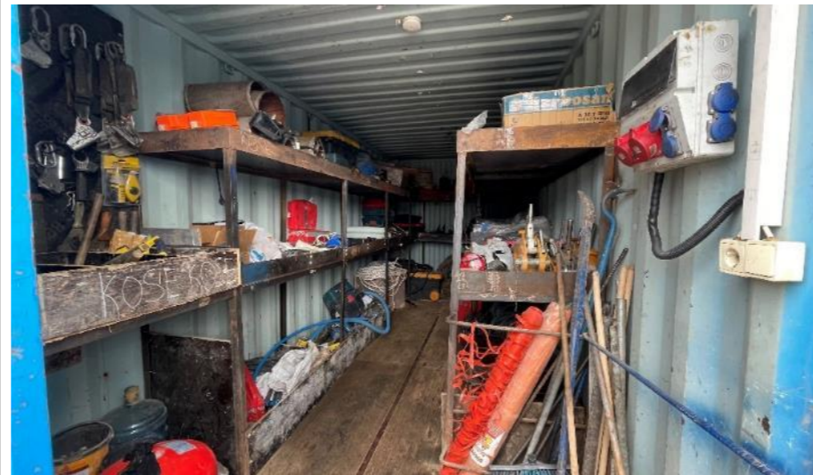
Figure 112. Material Warehouse in the Ağın Construction Site
