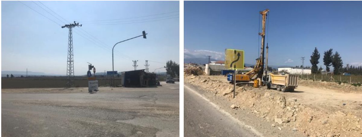
Figure 59. Antakya/Reyhanlı/Cilvegözü State Highway
