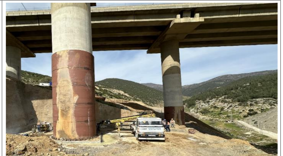
Figure 97. Working Area in the activity area of Başpınar Viaduct
