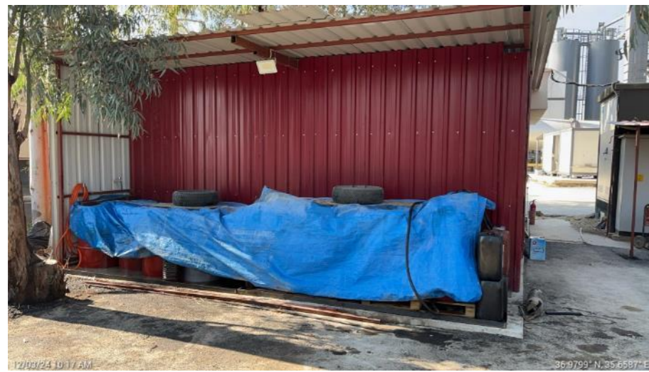
Figure 89. Chemical Storage Area in Ceyhan Const.&Accommodation Site
