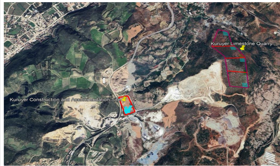
Figure 64. Kuruyer Limestone Quarry
