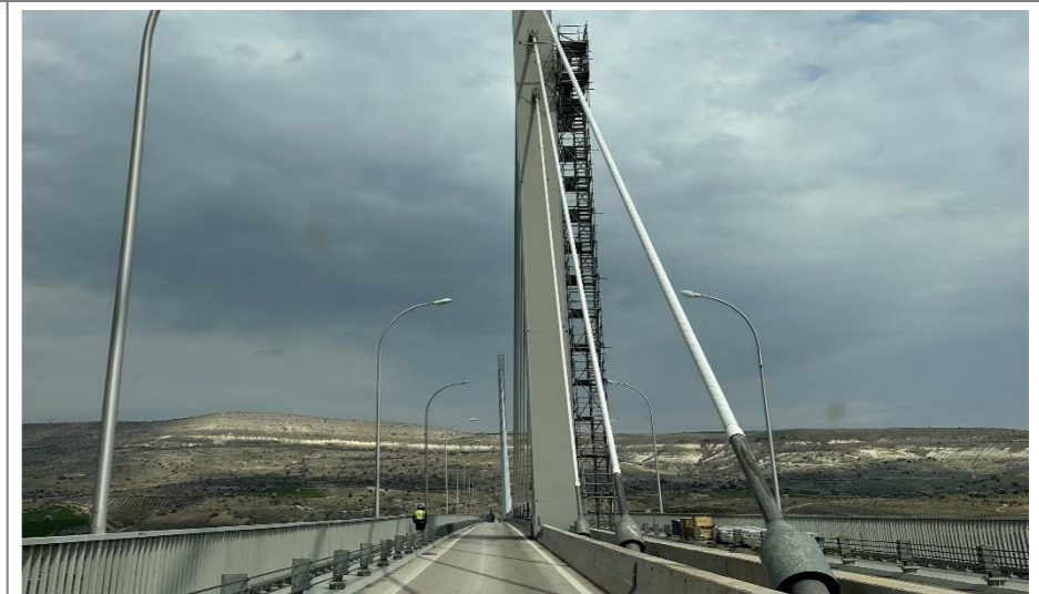
Figure 118. The scaffold set up at the Ağın Bridge
