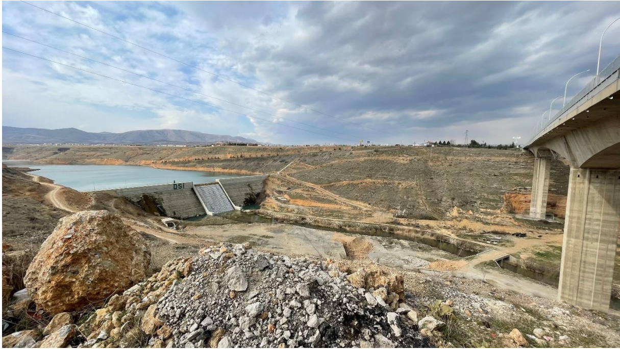
Figure 104. Yeşilvadi Reservoir and Beylerderesi Stream under the Beylerderesi Bridge
