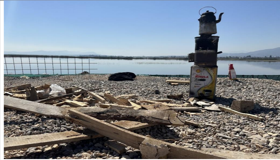
Figure 52. Non-conformity at the Hatay Airport Road Construction Site
