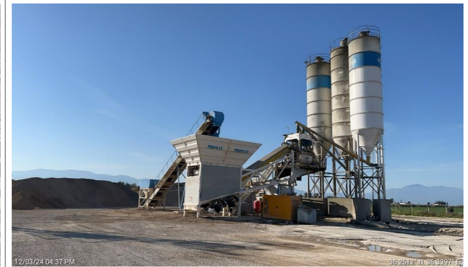
Figure 65. Concrete Plant used for Bridge Construction in Demirköprü
