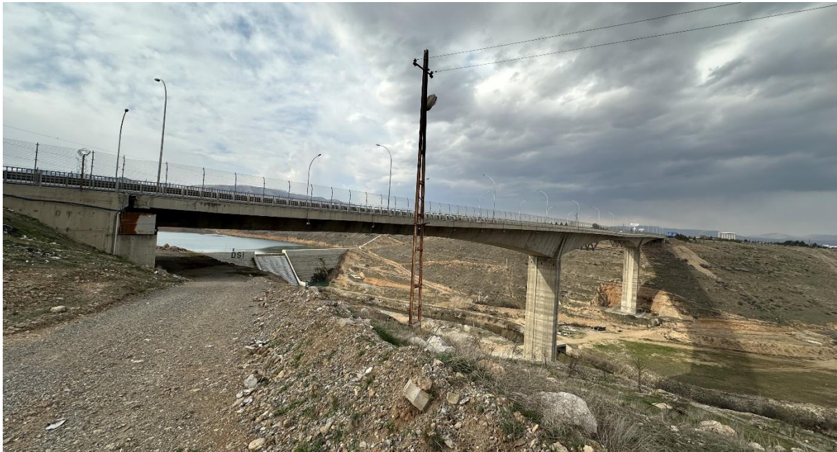
Figure 102. View of The Beylerderesi Bridge
