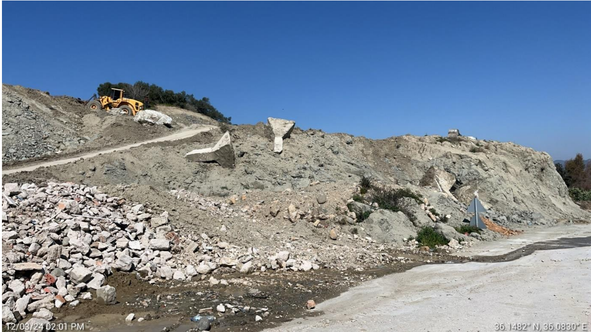
Figure 14. Landslide Removal Works
