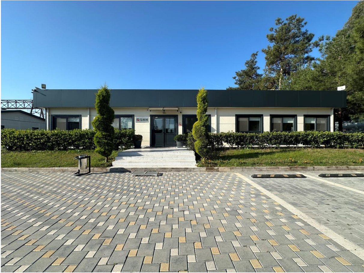
Figure 73. Ceyhan Construction and Accommodation Site - Offices
