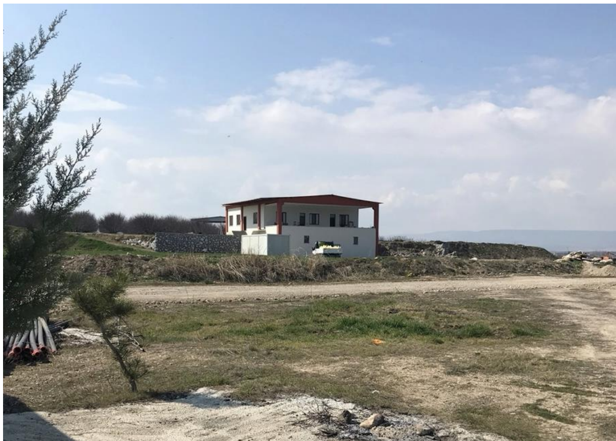
Figure 108. 2-storey house structure in the Tohma Camp Site Parcel
