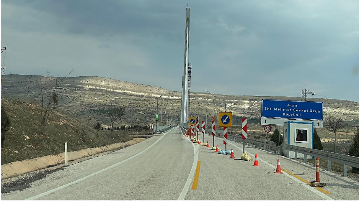
Figure 106. General View of Ağın Bridge -1
