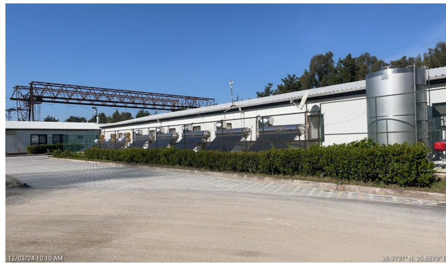
Figure 84. Solar Panels in Ceyhan Construction and Accommodation Site
