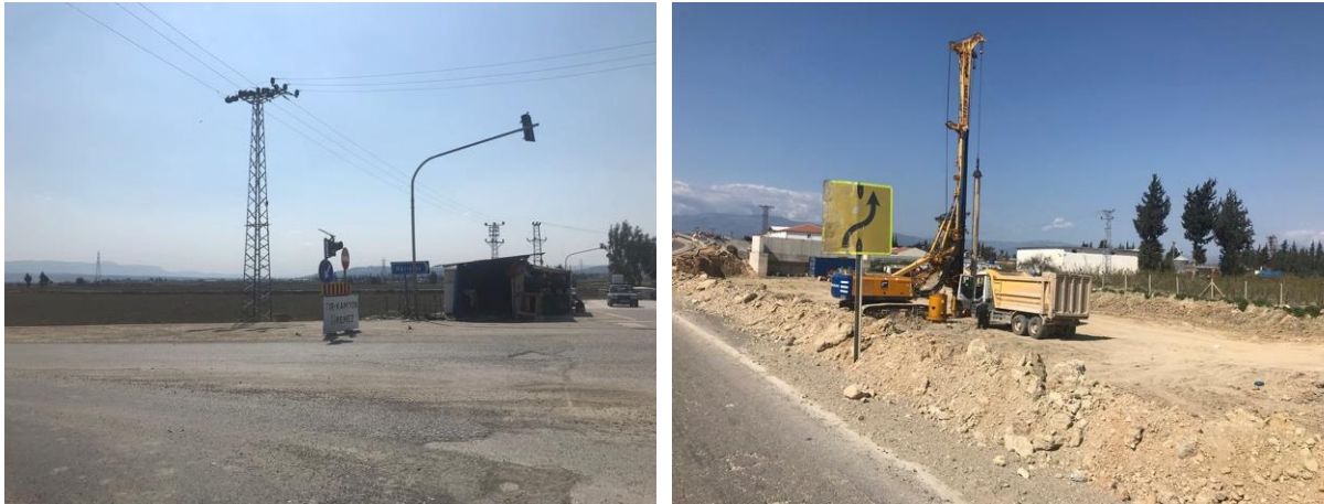
Figure 57. Antakya/Reyhanlı/Cilvegözü State Highway
