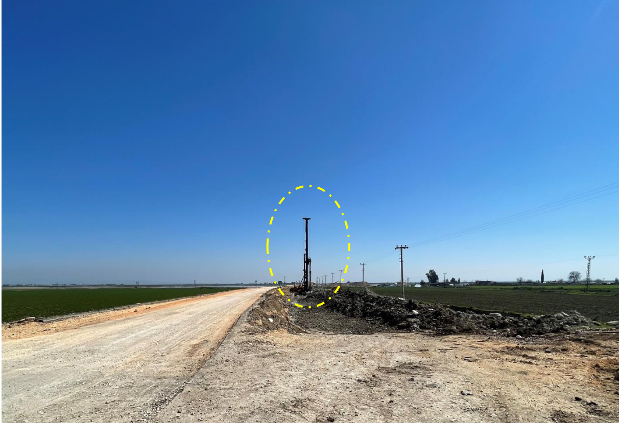
Figure 35. Deep Soil Mix (DSM) Machines on-site
