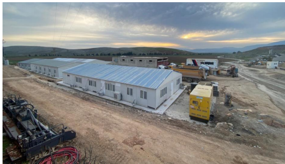
Figure 36. Kizilkaya Construction and Accommodation Site
