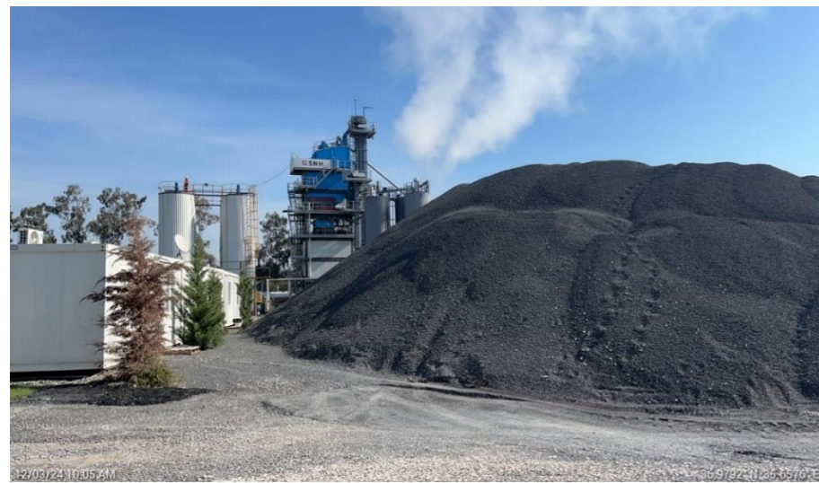
Figure 78. Asphalt Plant in Ceyhan Construction and Accommodation Site
