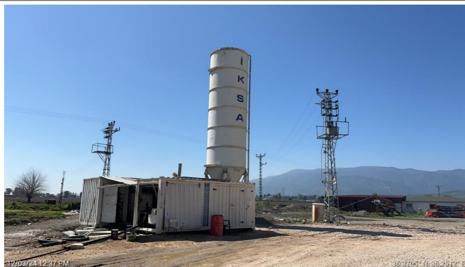
Figure 39. Deep Soil Mixing Station-1 at the Hatay Airport Road
