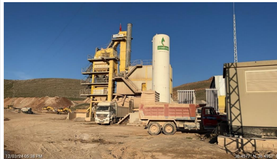
Figure 37. Asphalt Plant in Kizilkaya Quarry
