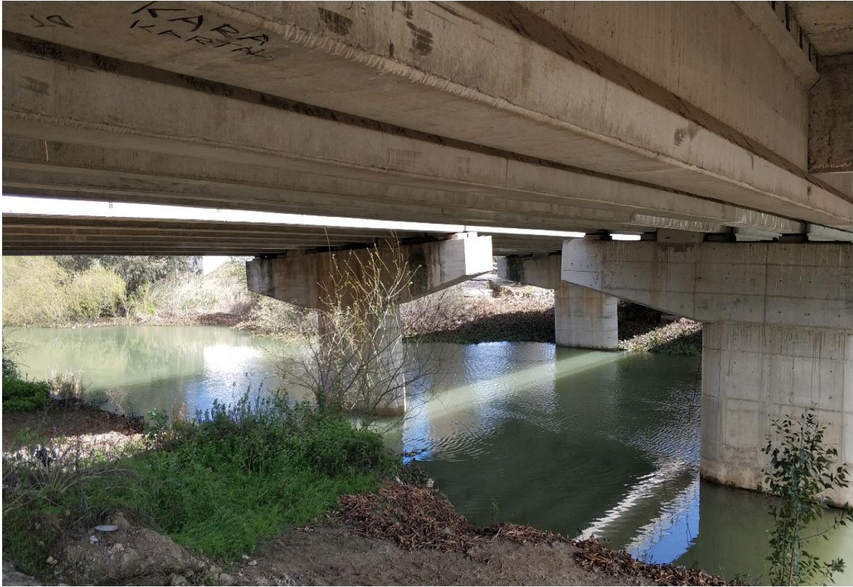
Figure 4. Damage on the Bridge Piers
