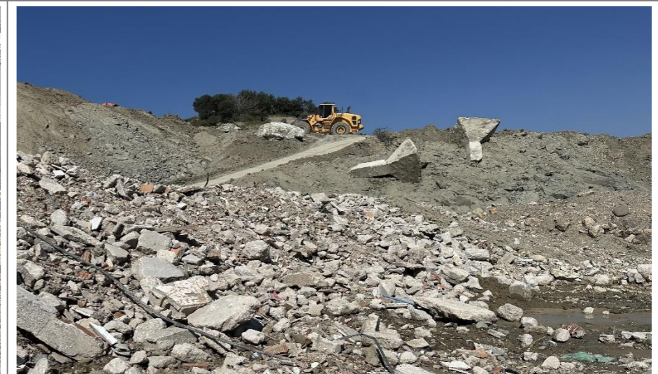
Figure 71. Landslide Area on the Antakya-Samandağ Road.
