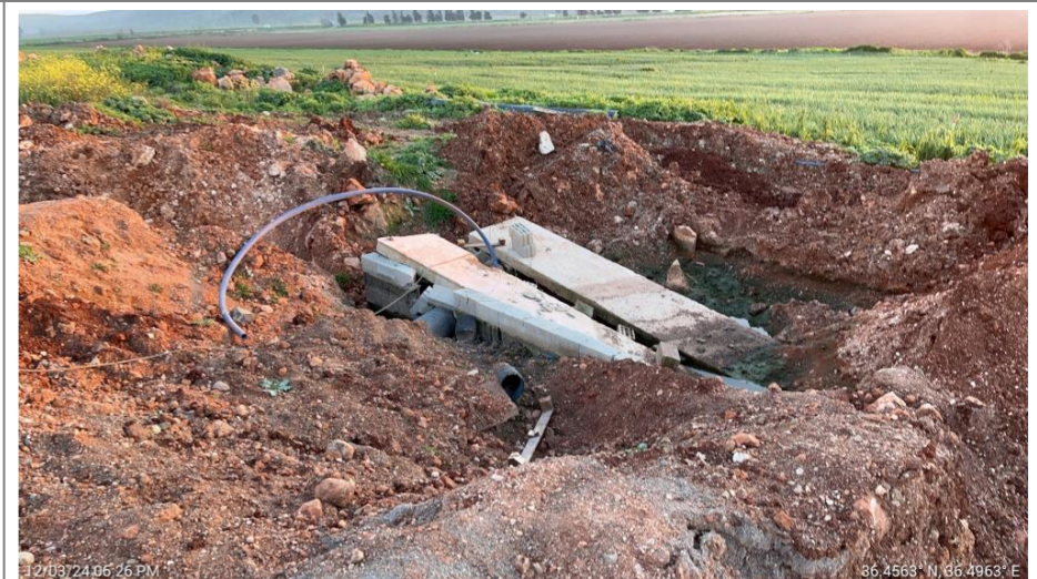
Figure 41. Old Septic Tank in the Kizilkaya Construction and Accommodation Site
