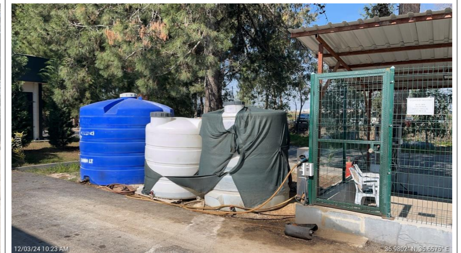
Figure 89. Storage Tanks in Ceyhan Construction and Accommodation Site
