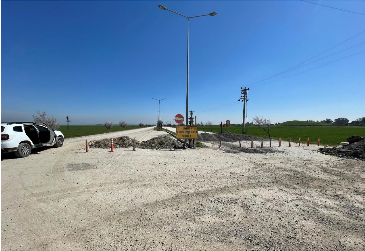
Figure 34. Entrance of the Sub-Project Construction Area
