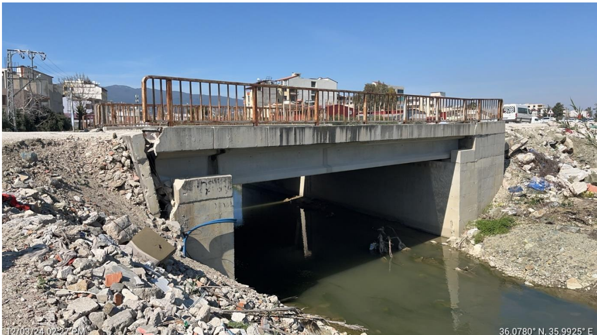
Figure 15. Bridge to be Reconstructed
