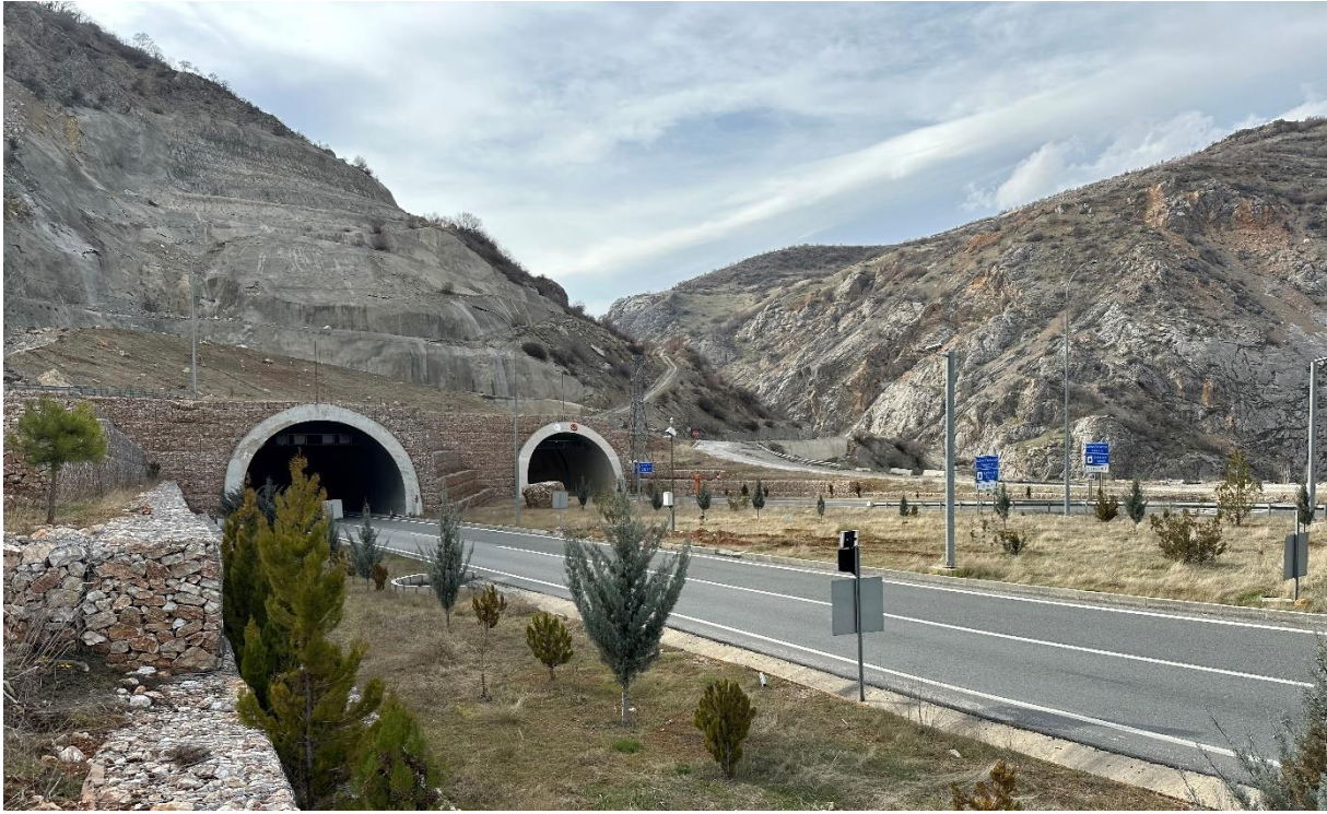
Figure 19. Erkenek Tunnel – Entrance Portal
