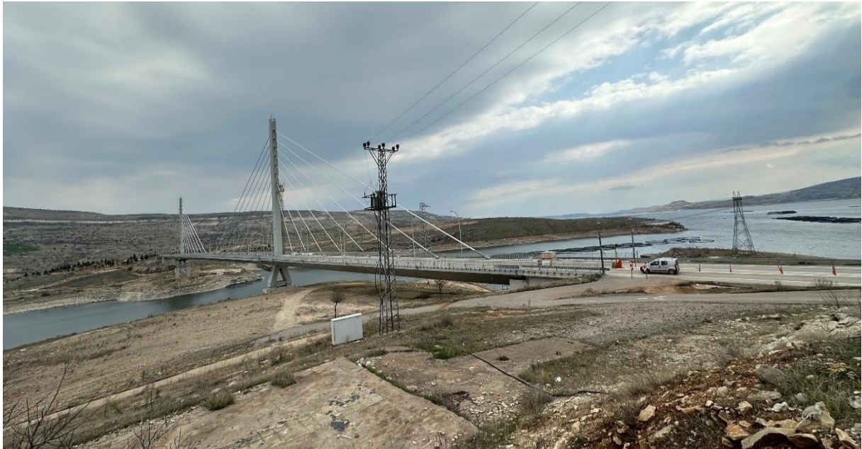
Figure 107. General View of Ağın Bridge -2
