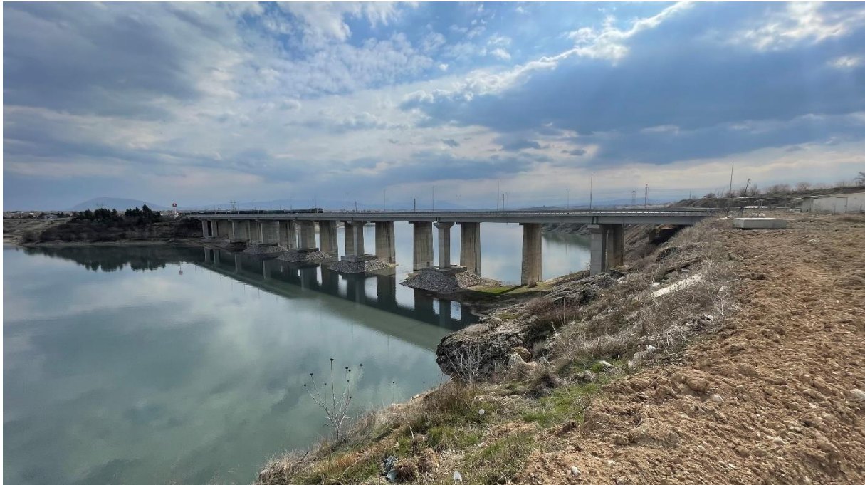
Figure 105. View of the Tohma Bridge
