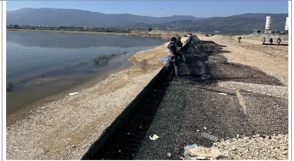
Figure 53. At the Hatay Airport Road Construction Site, Working at Heights
