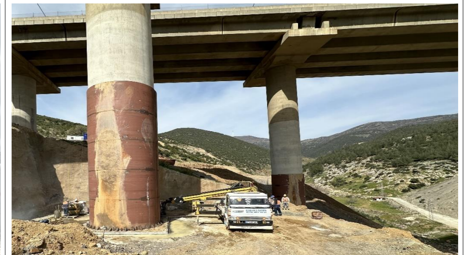
Figure 95. Working Area in the activity area of Başpınar Viaduct
