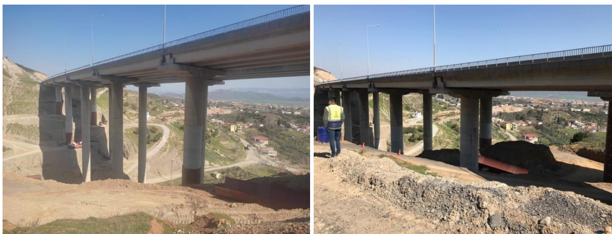
Figure 77. Başpınar Village and Başpınar Viaduct
