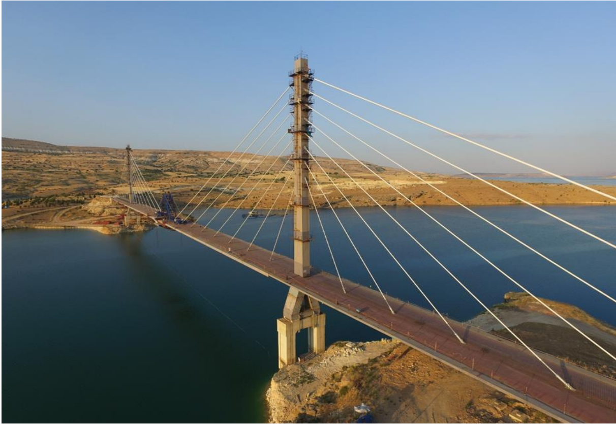
Figure 27. General View of Ağın Bridge
