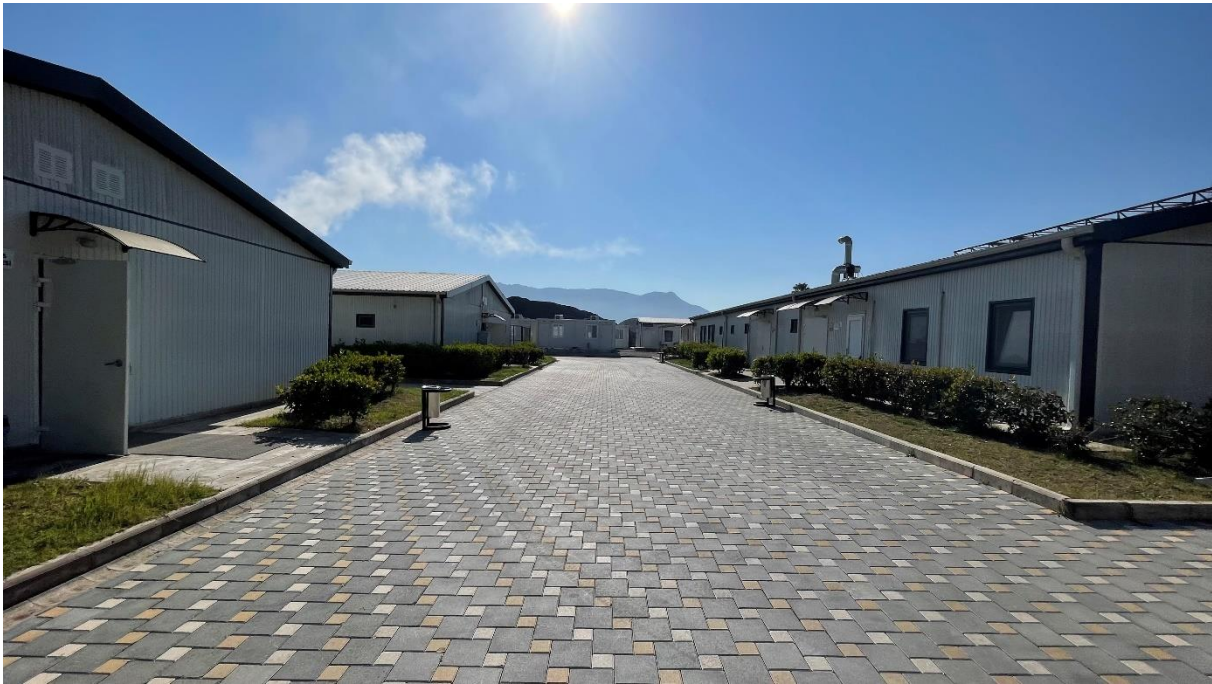
Figure 74. Ceyhan Construction and Accommodation Site - Accommodation Area
