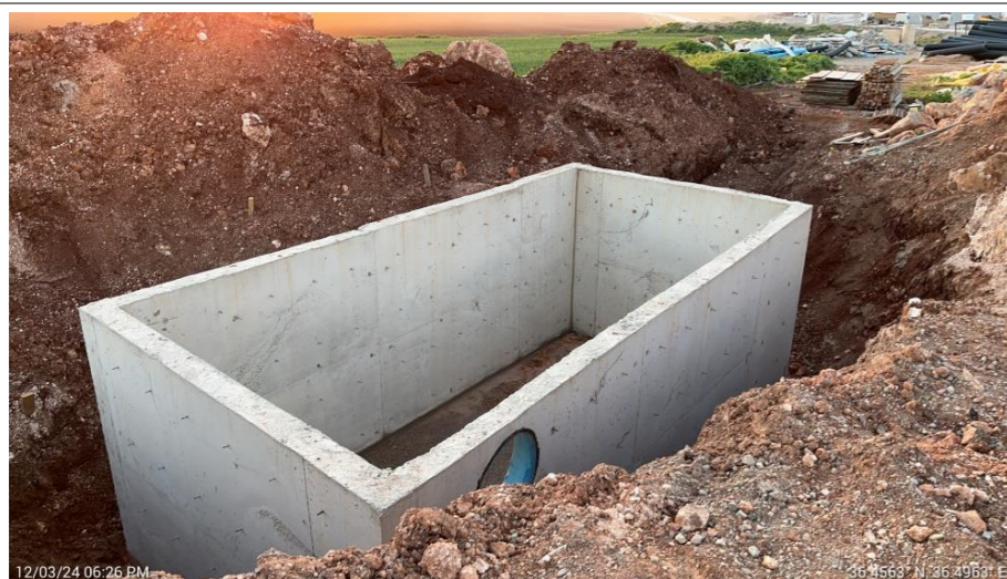
Figure 42. New Septic Tank in the Kizilkaya Construction and Accommodation Site
