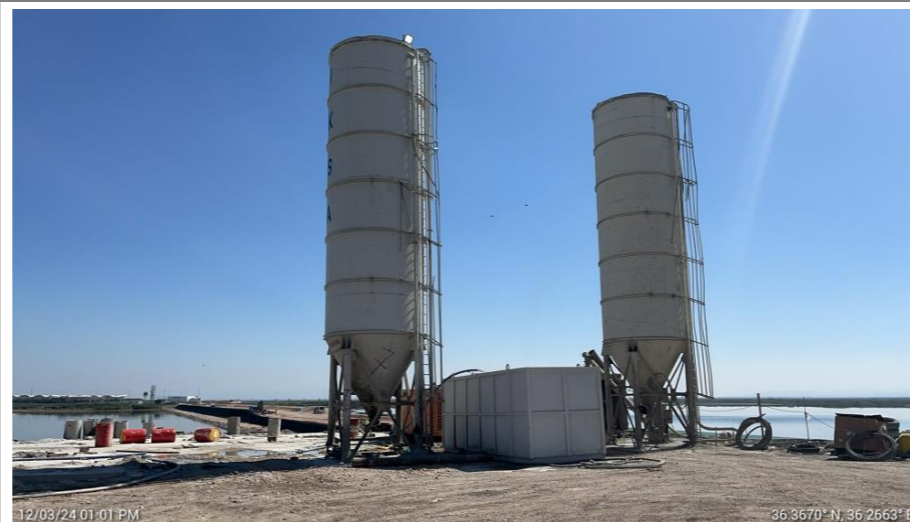
Figure 40. Deep Soil Mixing Station-2 at the Hatay Airport Road
