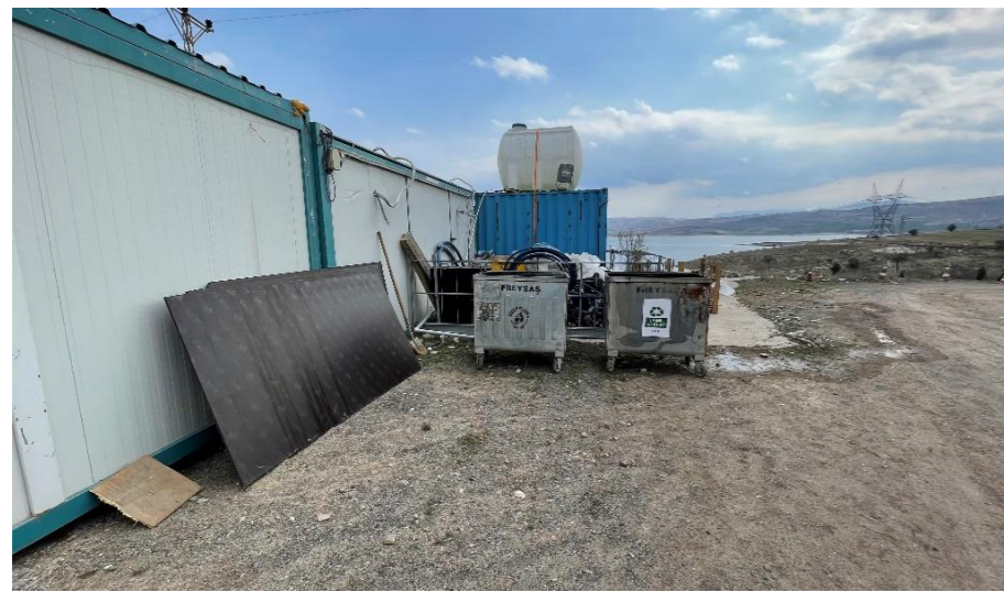
Figure 110. Domestic Waste Containers in the Ağın Construction Site
