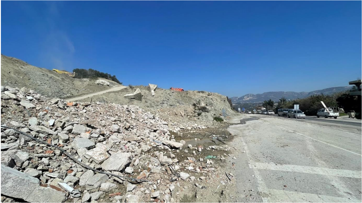
Figure 58. Landslide Removal Works at the Project Site
