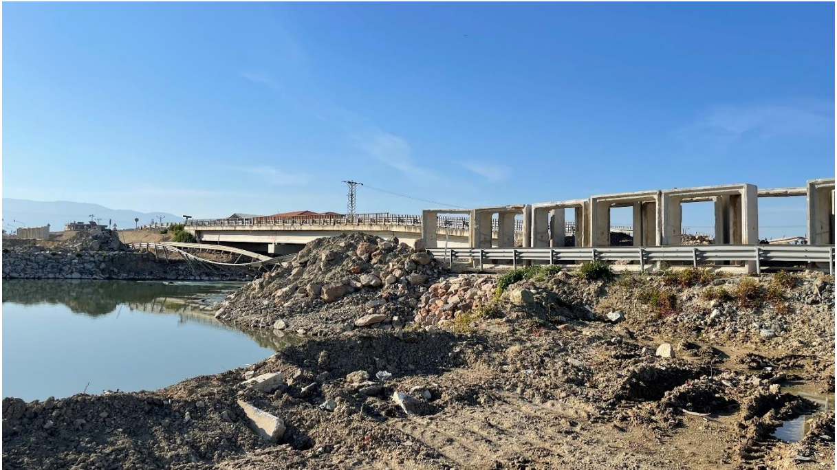
Figure 54. Demirköprü Bridge Construction Area
