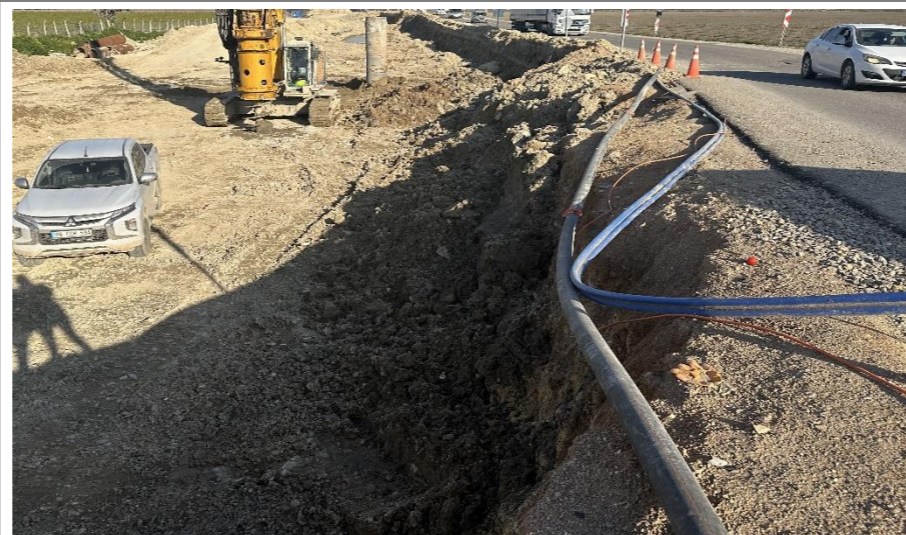
Figure 70. Antakya-Reyhanlı Road Construction Area
