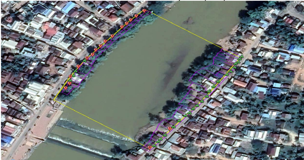
Figure 2.3: Barrage footprint (yellow), relocated AHs (green), affected other assets (red) and public land used as residential parcels (violet)
