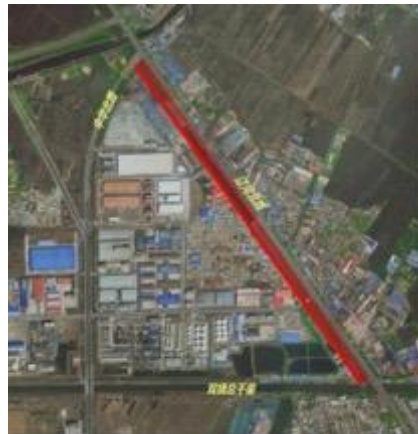
Figure 3-24 Satellite map of the green areas on both sides of the Goupan Canal
