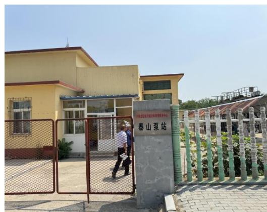
Field visit to Taishan Pump Station
