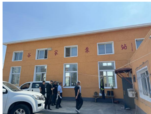
Field visit to Gujia Pump Station
