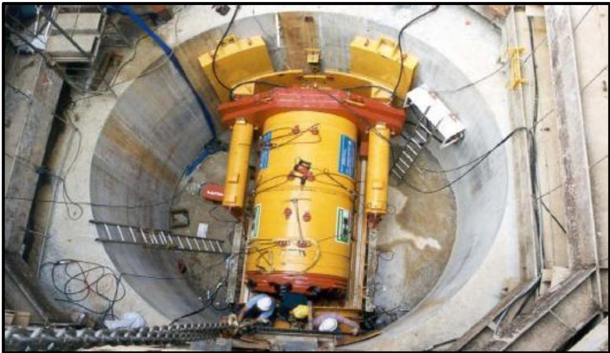
**Figure 3.6: A Typical Drive Shaft Arrangement with MTBM Lowered in the Shaft**
