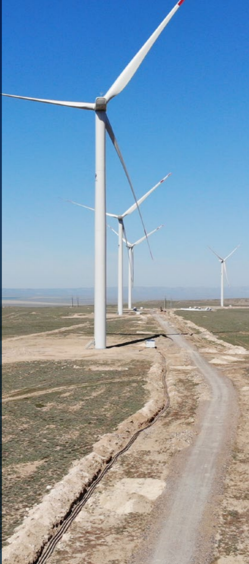
Zhanatas Wind-Power Station LLP 2021
